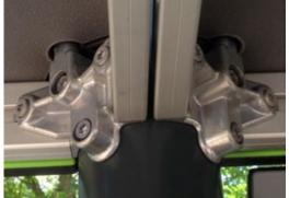
All decks are supported by unique designed aluminium profiles with multiple attachment options by usage of pressure moulded aluminium connectors. The HPL decks with a thickness of 17.8 mm with a very high wearing strength and a unique KOMPAN non skid surface texture.
